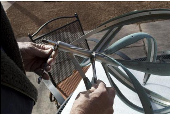
Use one of the two 9/16" wrenches on the top middle nut to keep them in place while you use the 1/2" wrench to loosen the long connector nut at the base of the sculpture.
